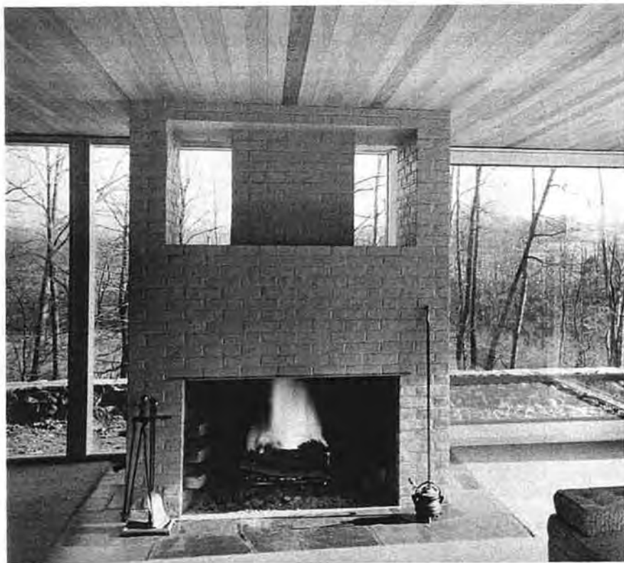
The Clark house. The all-brick fireplace features a projecting lintel over the firebox. The lintels supporting the upper band of brick are apparent from below.
