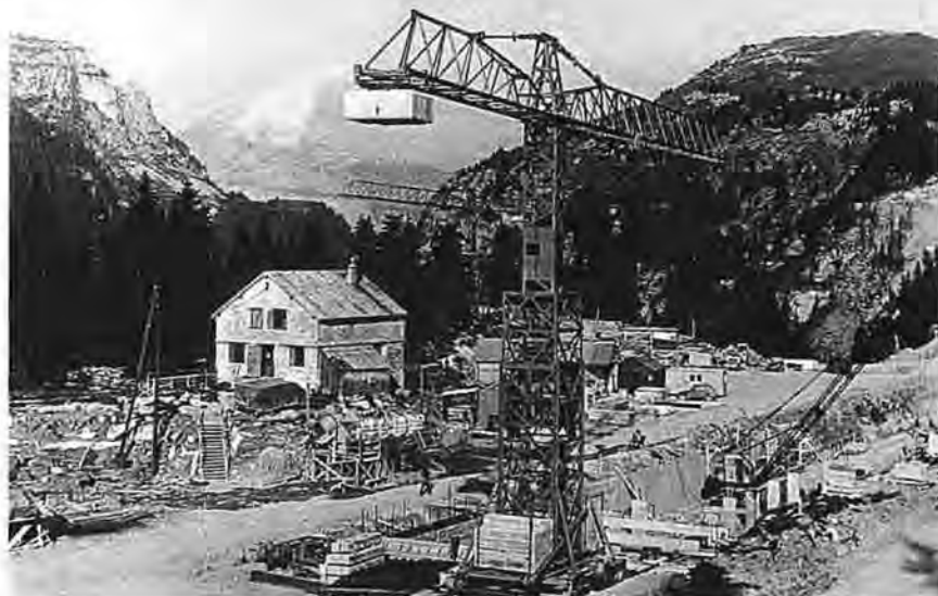
Flaine, 1961. The alpine shelter, Fédération, was still standing at the start of construction.
