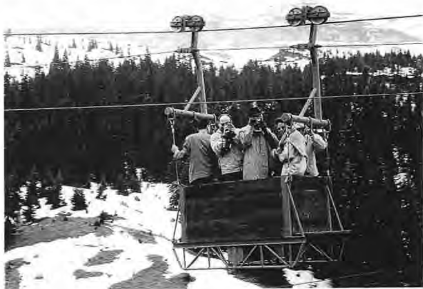
The design team riding the work gondola to the Grandes Platières, Flaine, 1966.
