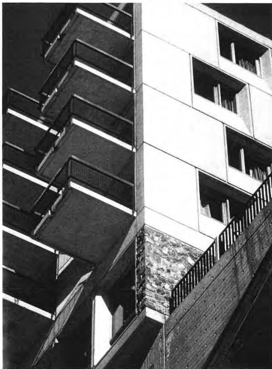
Hôtel Le Flaine. Non-load-bearing windows, balconies, and facade panels are stacked on the left to create a "fabric" of mullions and voids; Breuer instinctively staggered the joints of the end wall to imply the masonry's ability to bear load.
